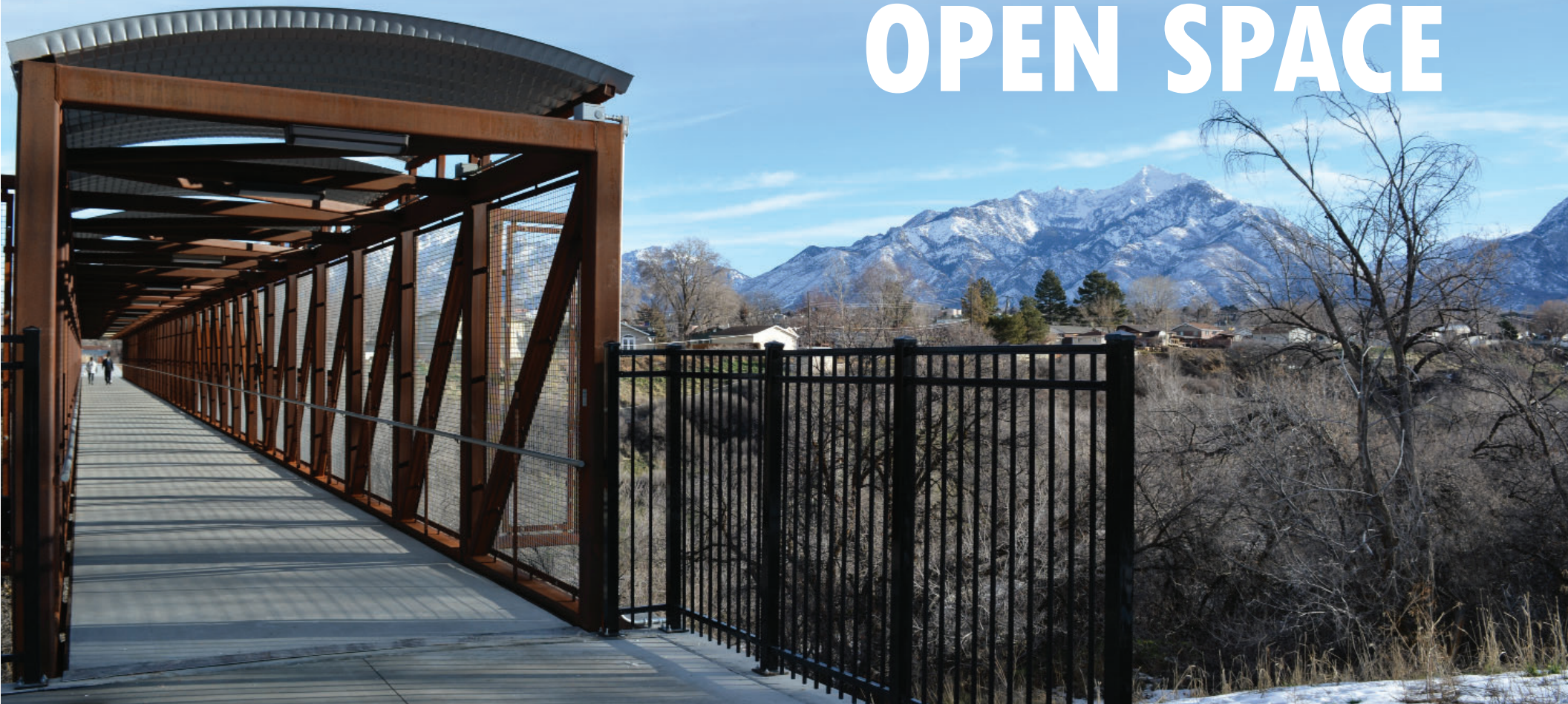
Bridge at Dimple Dell Park
