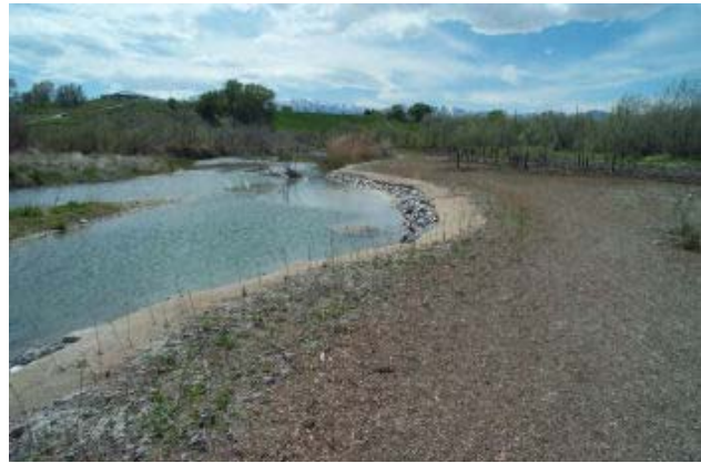
Riverbend restoration site along the Jordan River after construction (2002)
