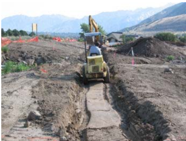
Excavation near Corner Creek, Lower Corner Creek Sub-Watershed
