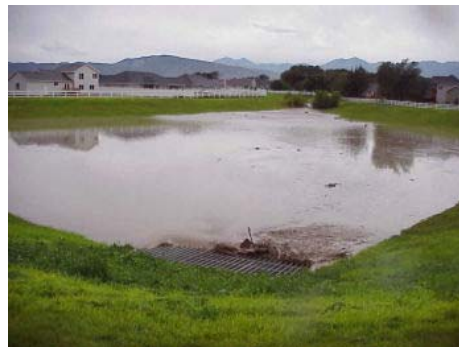
Detention pond on Midas Creek during flood event
