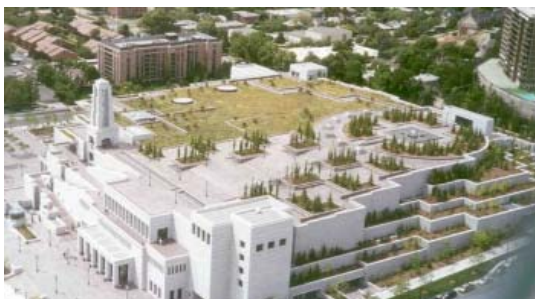
Green roof on Latter-Day Saint Conference Center, Jordan River Corridor Sub-Watershed
