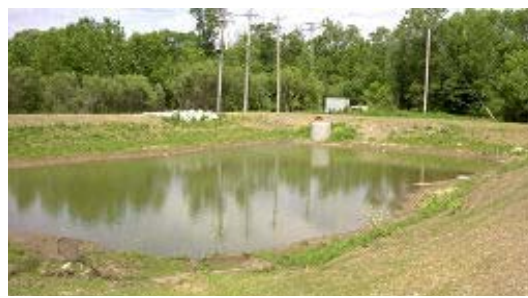
Example of a Sediment Basin
