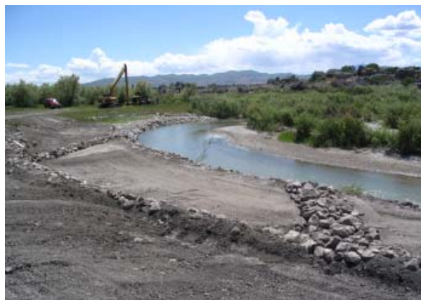
Jordan River ecosystem restoration project at 11400 South, Jordan River Corridor Sub-Watershed
