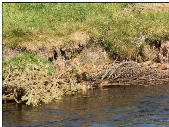
Example of Revetment
