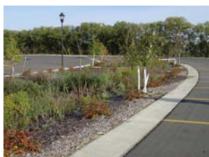
Example of Bioretention Cells
