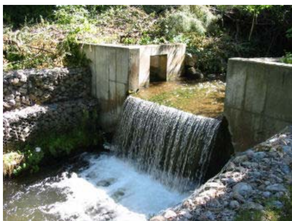
Diversion structure on Mill Creek, Lower Mill Creek Sub-Watershed
