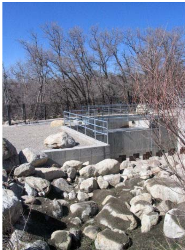
Drinking water diversion off of Willow Creek, Lower Willow Creek Sub-Watershed
