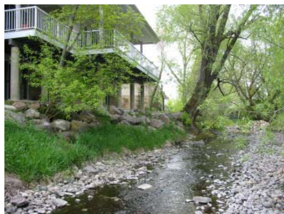
Residence adjacent to Little Cottonwood Creek, Lower Little Cottonwood Creek Sub-Watershed
