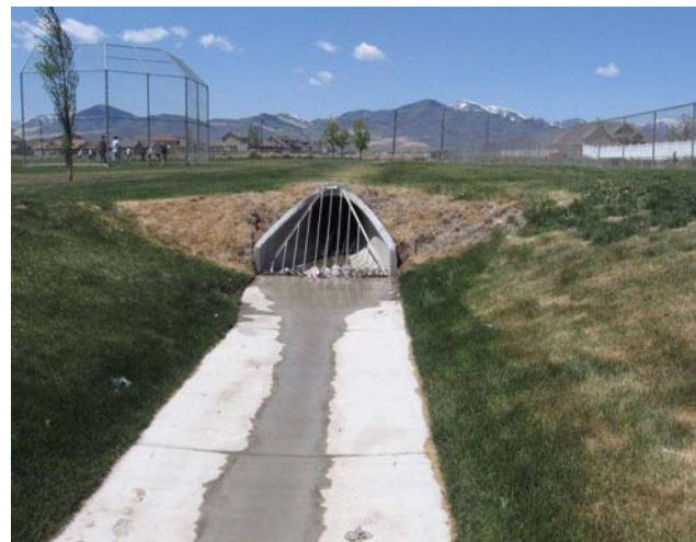
Barneys Creek emerging from culvert through West Hills Middle School campus.
