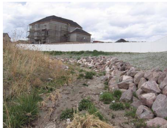
New residential development along Midas Creek in Riverton.
