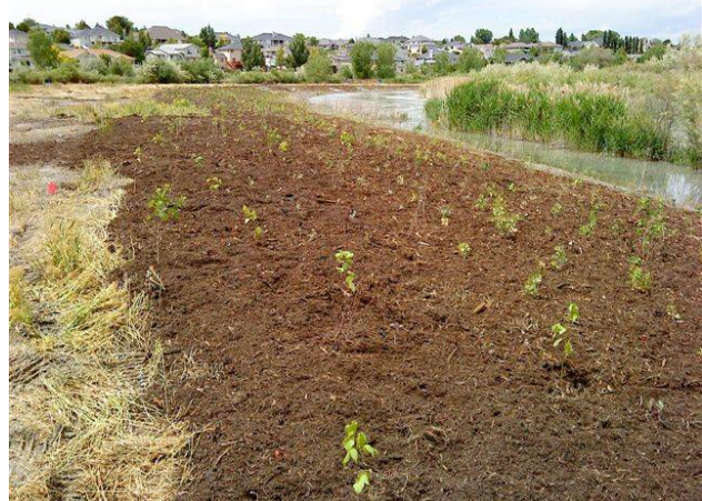
Example of before (above) and after (right) river restoration project completed in 2009 using Emergent Bench model along the Jordan River. This site in Riverton will be irrigated for 2 years to establish vegetation.
