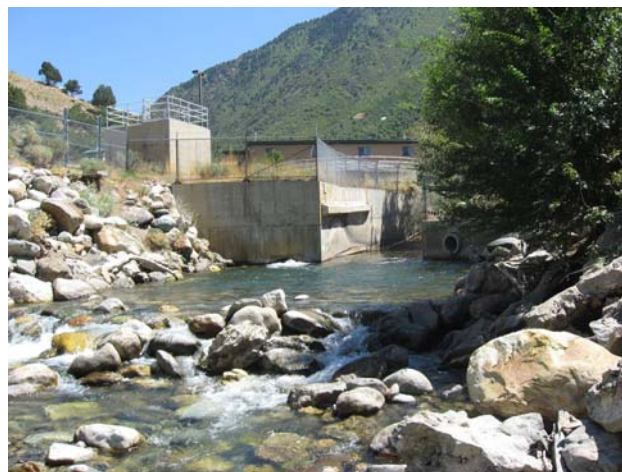
Big Cottonwood Creek below the water treatment plant near the canyon mouth.
