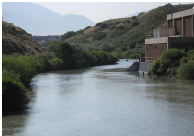
Jordan Valley Water Conservancy District's Jordan Narrows Pump Station in Bluffdale.
