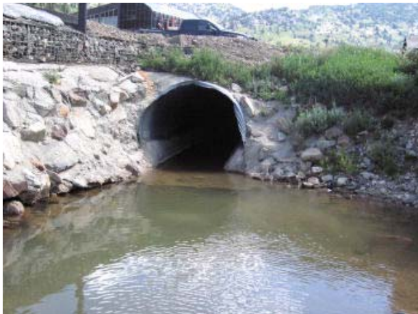
Little Cottonwood Creek Culvert, Upper Little Cottonwood Creek Sub-Watershed
