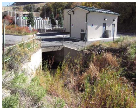
Parley's Creek Diversion Facility
