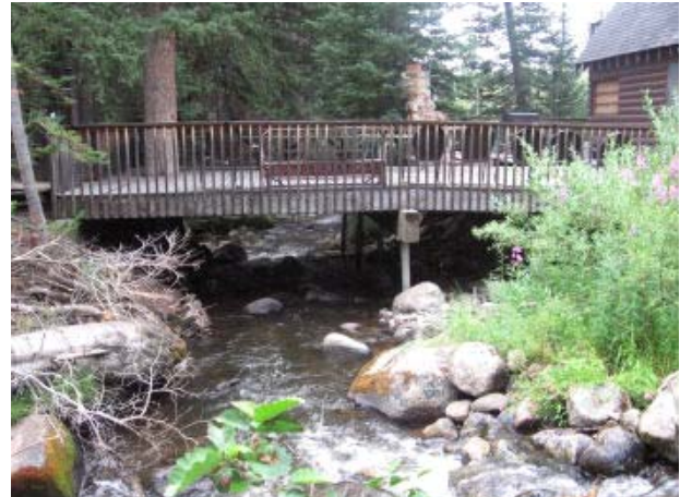
Foot Bridge over Big Cottonwood Creek, Upper Big Cottonwood Creek Sub-Watershed
