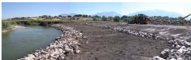
Panorama of a Jordan River Channel Restoration Site
