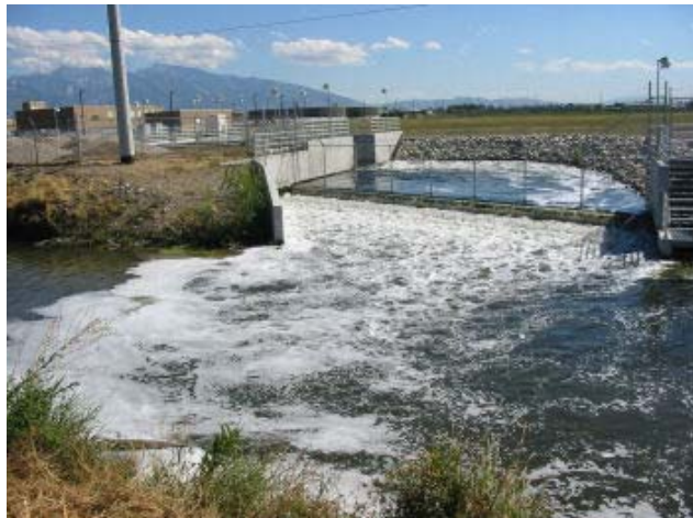
Central Valley Water Reclamation Facility discharge to Mill Creek, Lower Mill Creek Sub-Watershed
