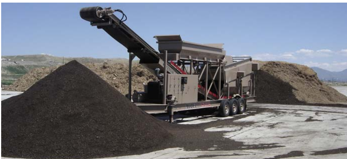
Central Valley Water Reclamation Facility biosolids compost product
