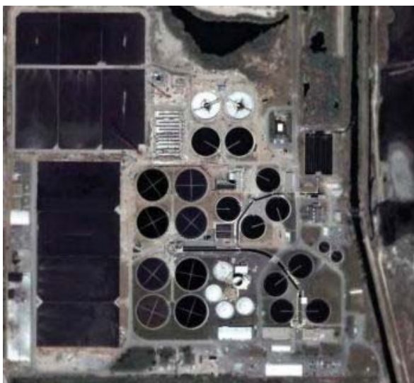
Wastewater Treatment Facility, Great Salt Lake Sub-Watershed
