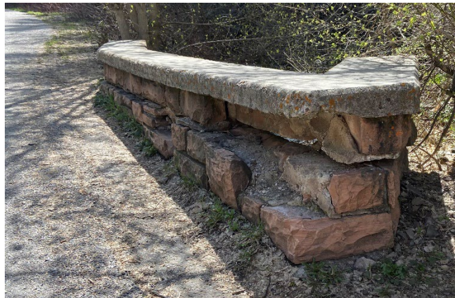
Figure 8. Stone Bridge 1 Wall
