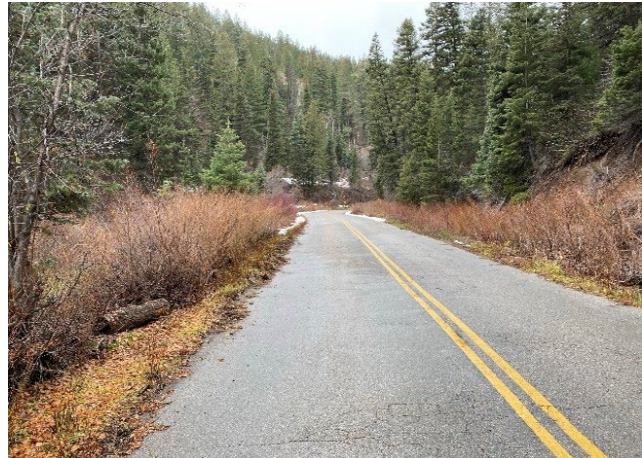
Figure 11. Typical Roadside View in Upper Mill Creek Canyon
