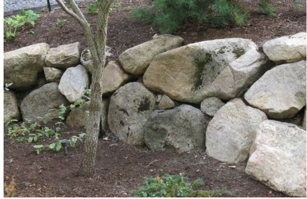
Figure 6. Example of a Rockery Wall
