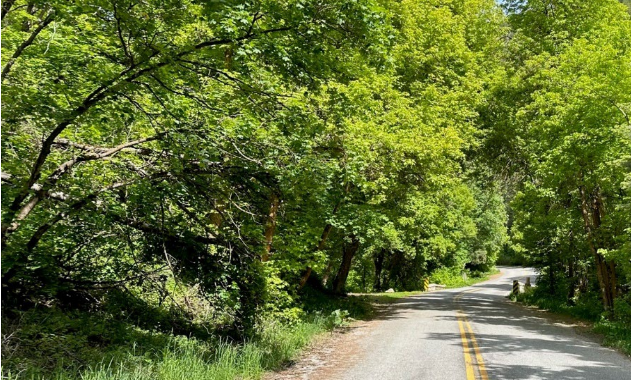
Figure 3. Road Narrowing at White Bridge
