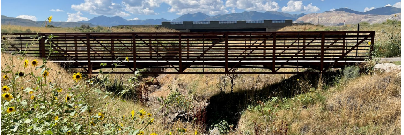
Midas Creek pedestrian bridge
