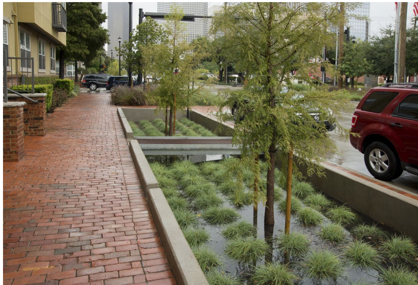
Rain gardens along an urban street in midtown Houston slow and filter stormwater runoff.
