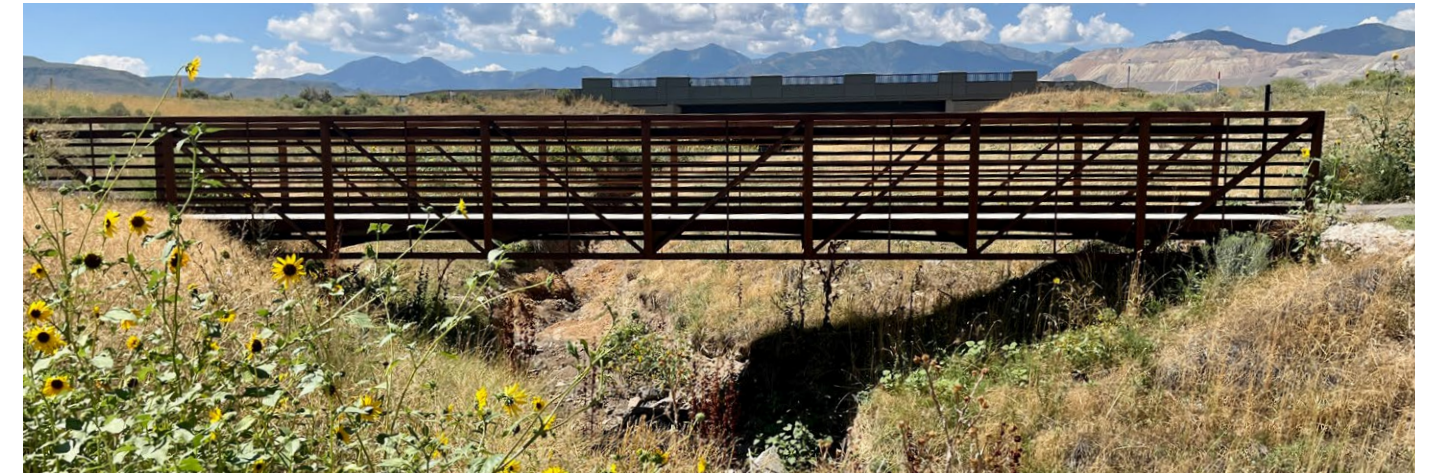
Midas Creek pedestrian bridge
