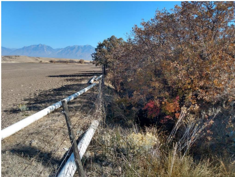
Photo 2-4 Butterfield Creek Channel that has been encroached by Farming Activities
