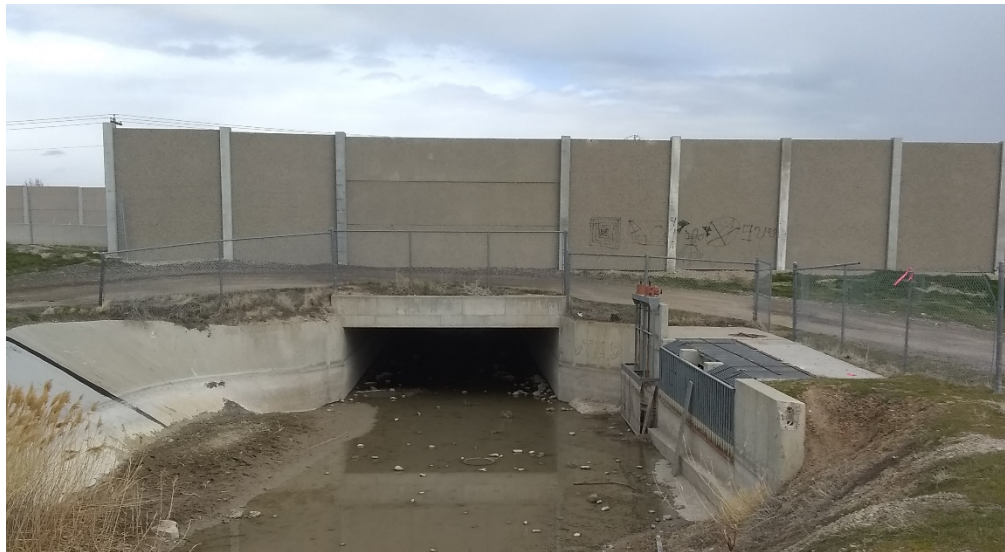
Photo 2-1 Overflow/Dump-Out Structure at Utah and Salt Lake Canal
