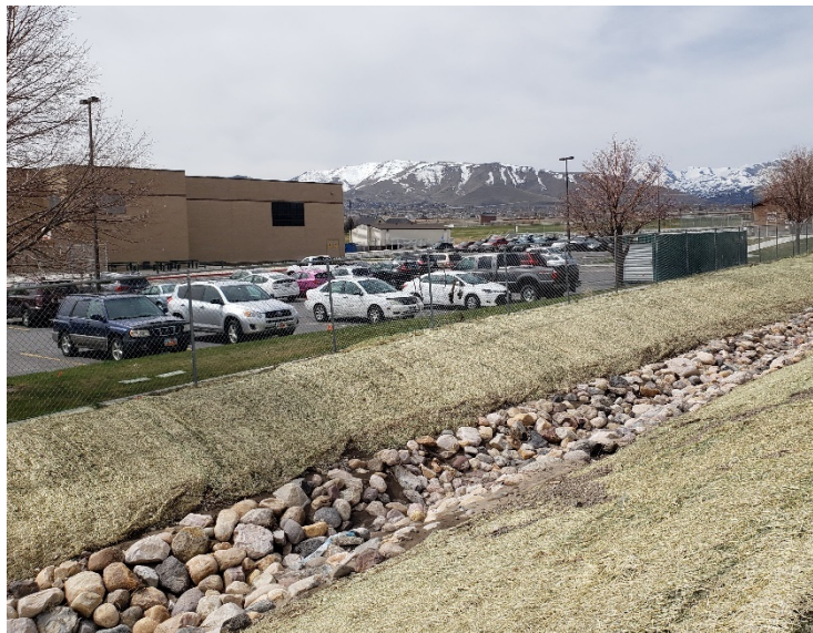
Photo 2-3 Uncertified Levee upstream of 4000 West adjacent to the South Hills Middle School
