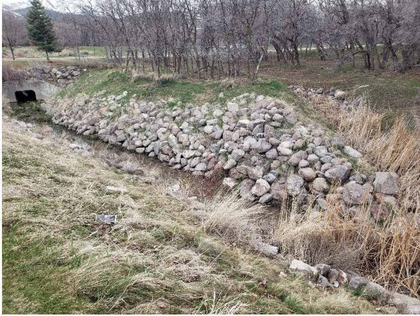
Photo 2-5 Rounded riprap upstream of Spring Canyon Drive (6090 West)
