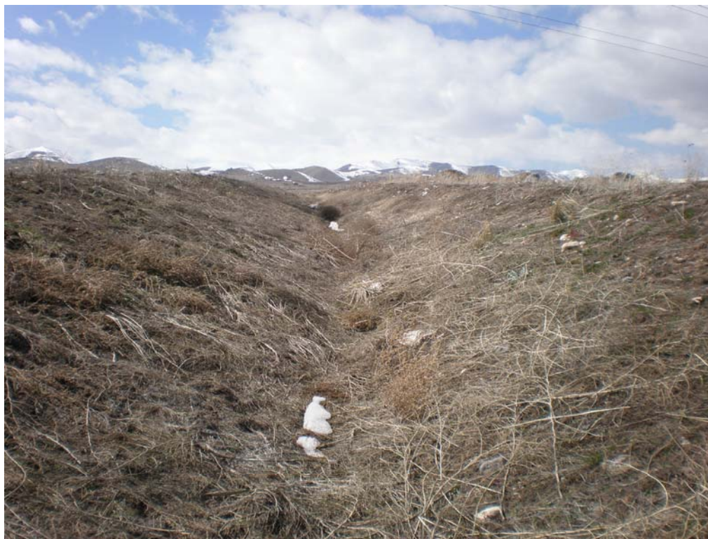
Figure 25. Man-made triangular channel in power station area, looking upstream
