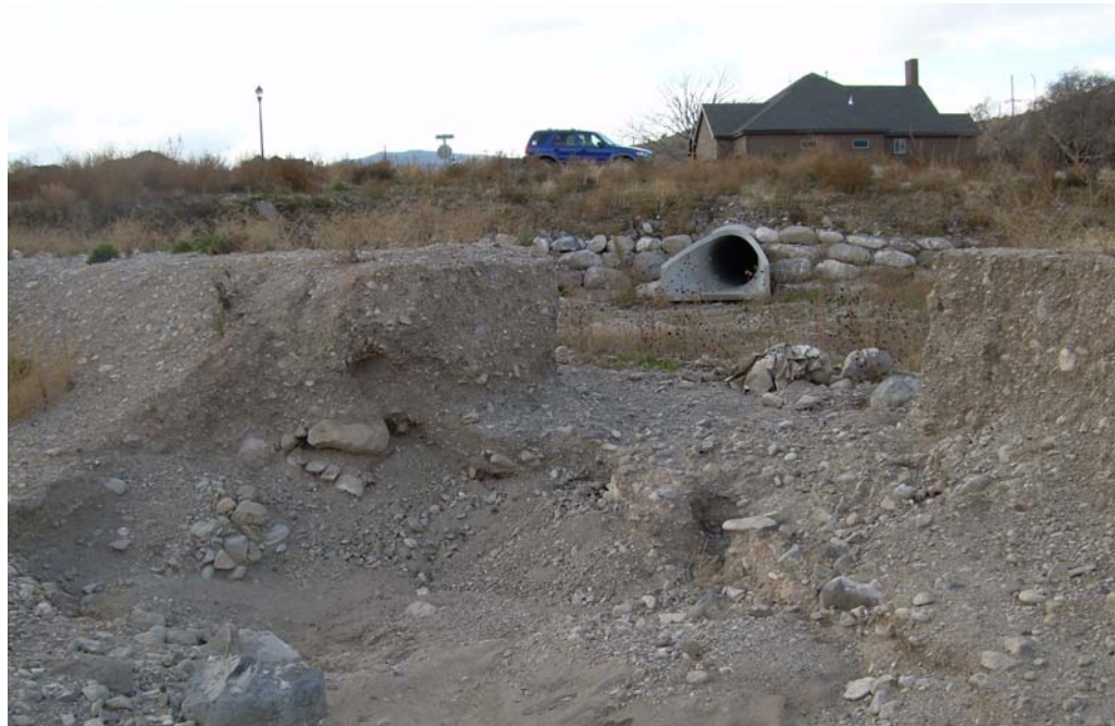
Figure 26. Parry Farms detention basin November 2007
