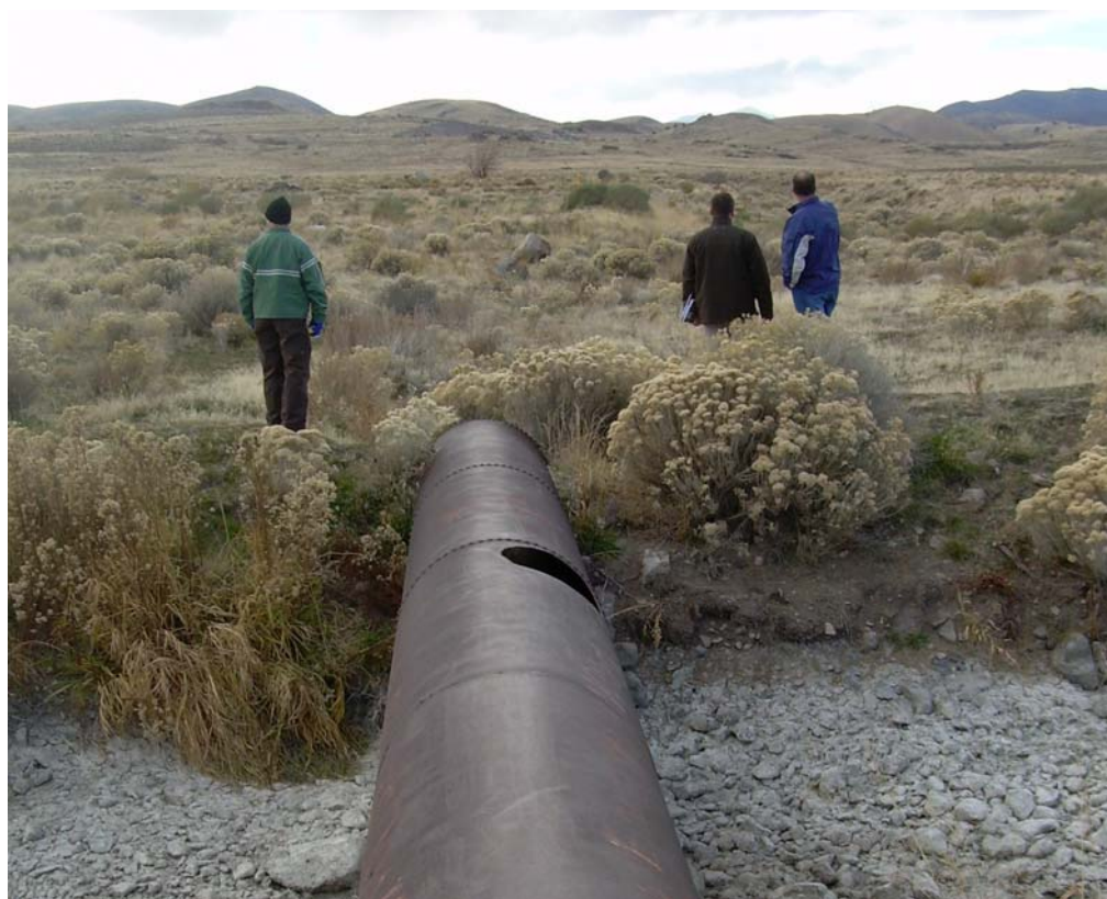
Figure 24. Looking upstream of the steel pipe crossing over the Provo-Reservoir canal
