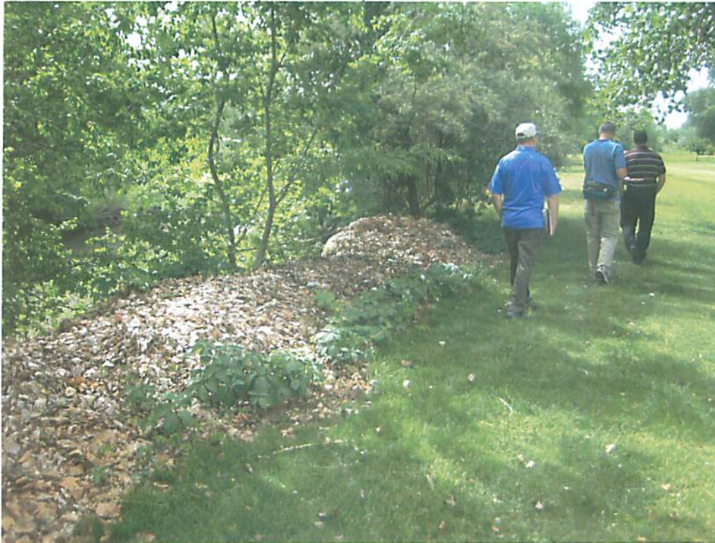
PHOTO 5 Leaf Debris Piles on the Levee Crest (river on the left)
