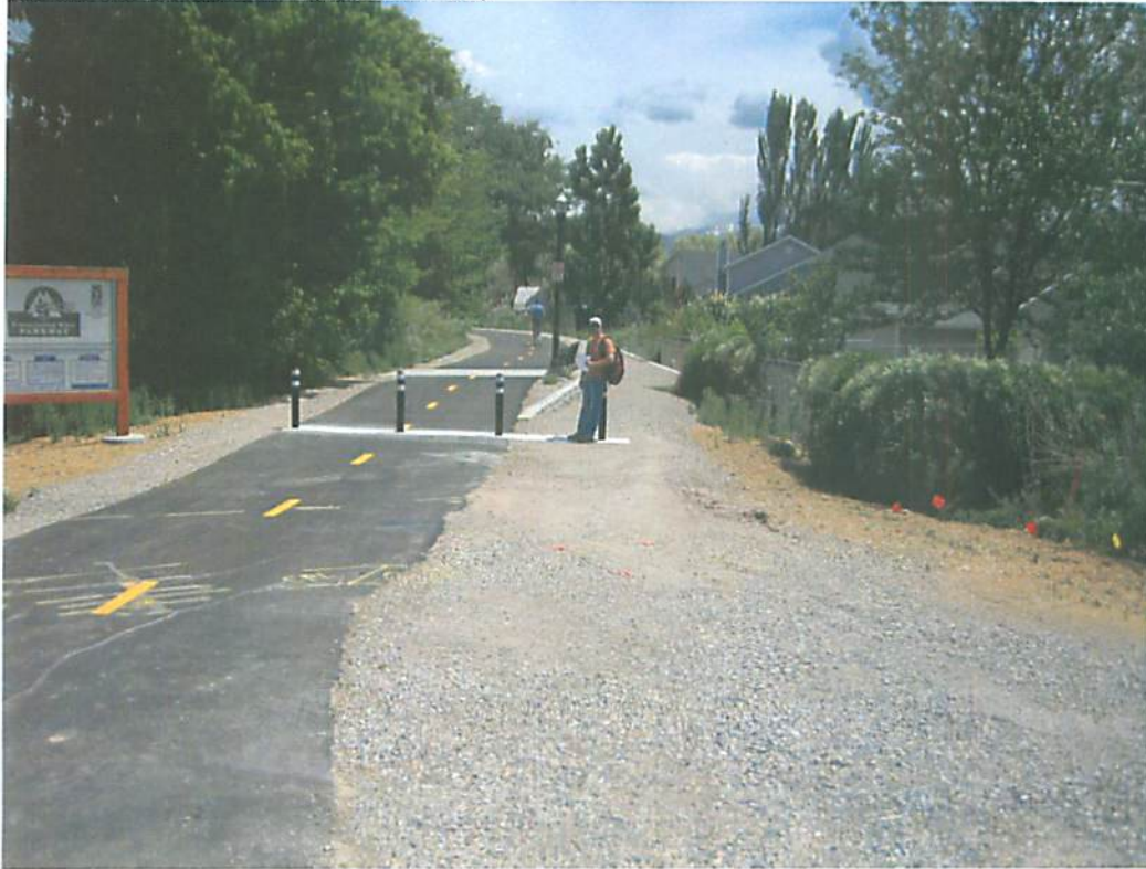
PHOTO 1 Paved Path on Levee Crest (river on the left)
