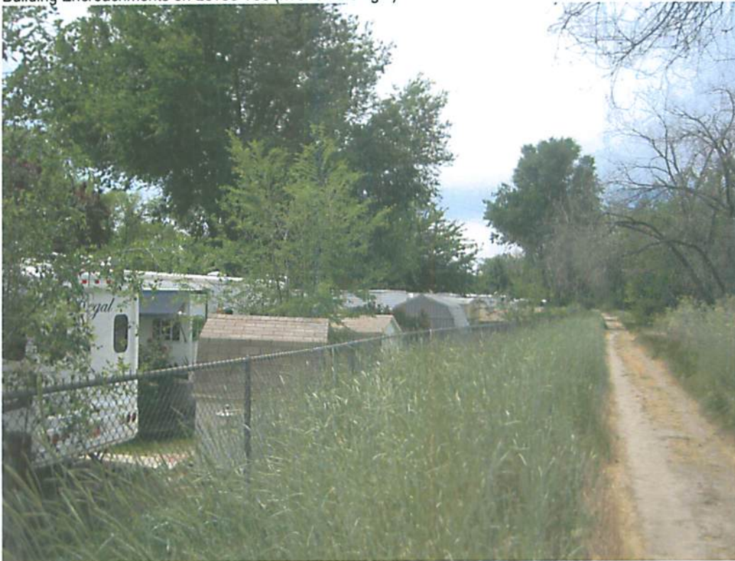
PHOTO 22 Building Encroachments on Levee Toe (river on the right)
