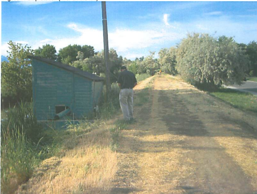
PHOTO 10 Irrigation Pump Station (river on the left)
