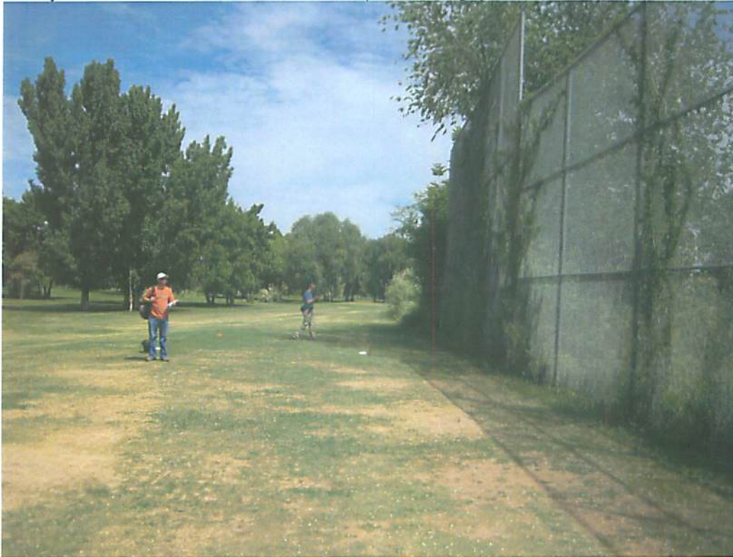
PHOTO 3 Fairway is Part of Levee, Fence on the Levee Crest (river on the right)
