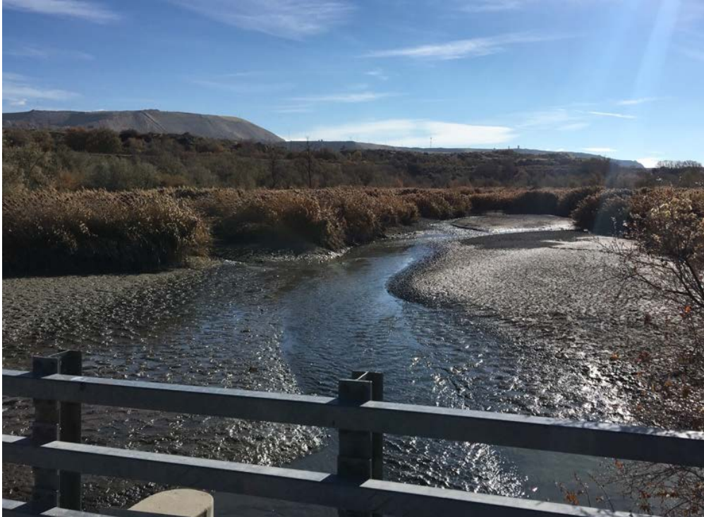
Photo 7: Sediment deposition upstream of the Joint Diversion
