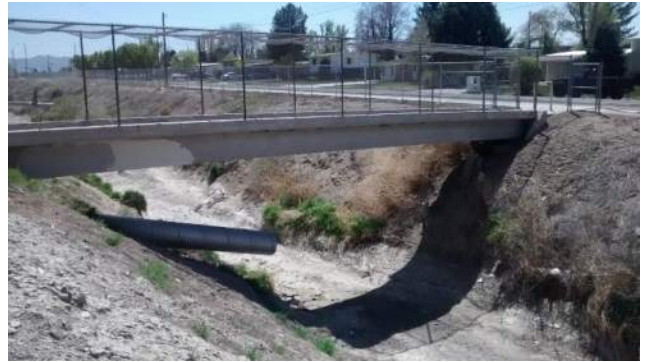
Pedestrian Bridge and Outfall at Approximately 4900 South
