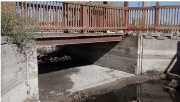
Pedestrian Bridge Immediately North of 7800 South near Gardner Village
