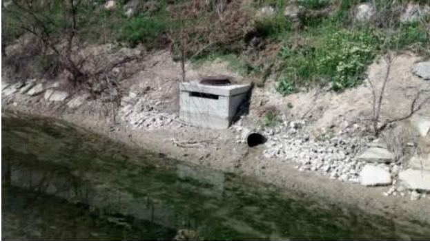
Outfall at Approximately 7400 South
