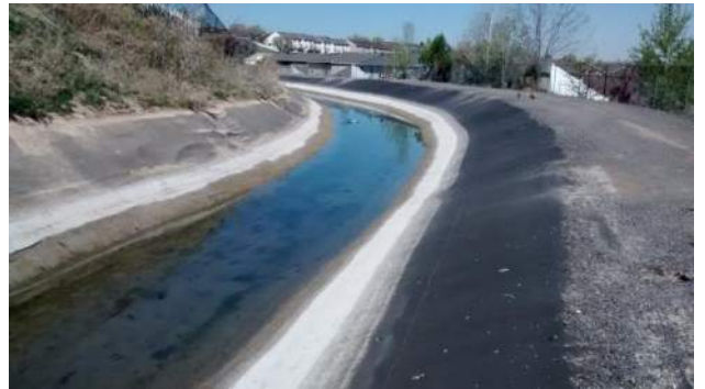
Canal Lining at Approximately 6800 South
