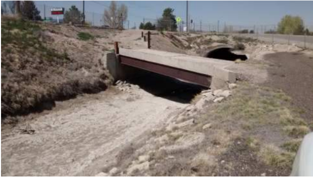
Maintenance Access Road Bridge and Culvert at Morning Vista Drive
