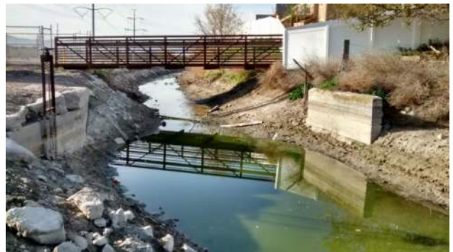
Pedestrian Bridge & Irrigation Turn out - Approximately 8600 South
