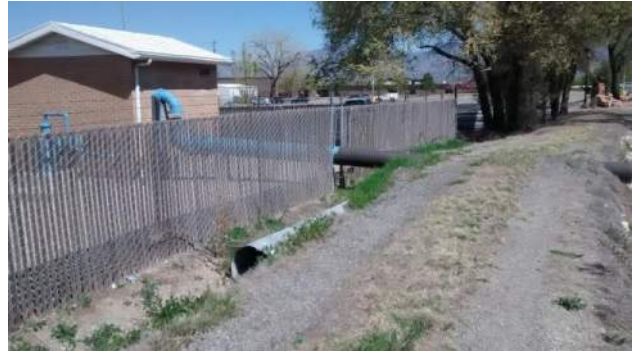
Pump Station at Approximately 1850 West
