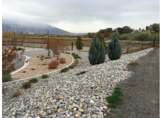
Trees on the Embankment - Approximately 8270 South
