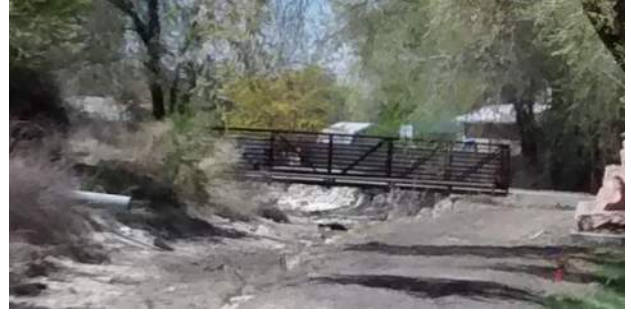
Pedestrian Bridge at Approximately 1800 West
