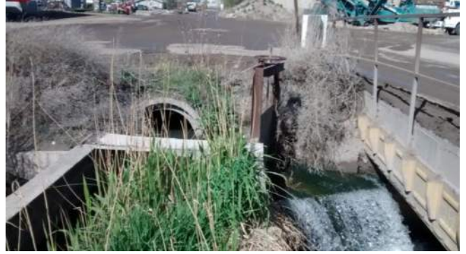
42 inch Outfall at approximately 7500 South
