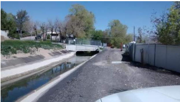
Monitoring Station and Winchester Street Culvert
