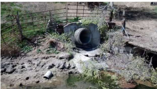
36 Inch Outfall at Approximately 6400 South
