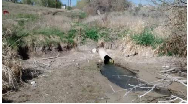
Spring Discharging into NJC at Approximately 7600 South
