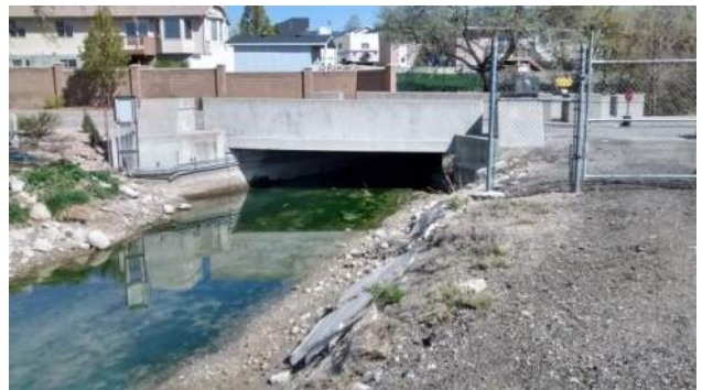
Culvert at 7500 South
