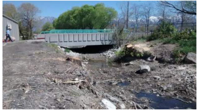
Pedestrian Bridge at Approximately 2100 West
