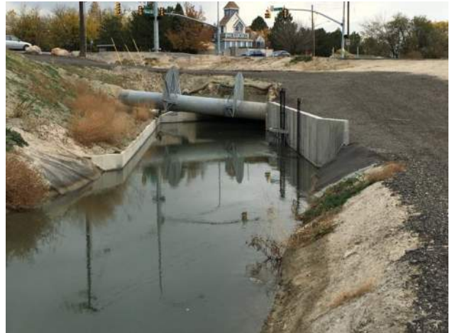
Storm Drain Overflow/Dump-out at 5400 South
