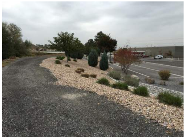
Trees on the Embankment - Approximately 8250 South
