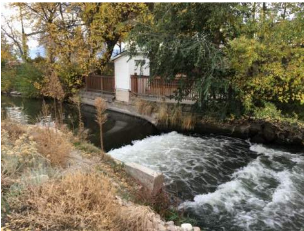
Concrete Flume Immediately North of 7800 South near Gardner Village
