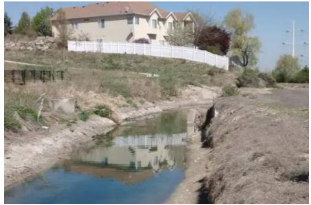
Utility Crossing at Approximately 7100 south
