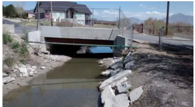
Bridge at Bullion Street
