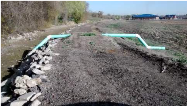
Pipe Penetration through the Embankment - Approximately 8370 South
