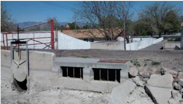
Overflow Structure at Approximately 2700 West
