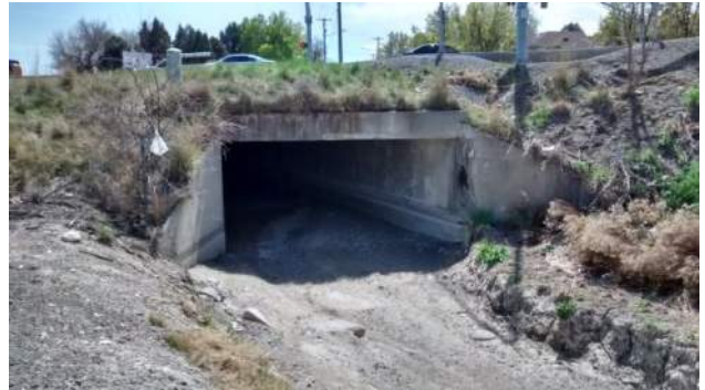
Culvert at 5400 South
