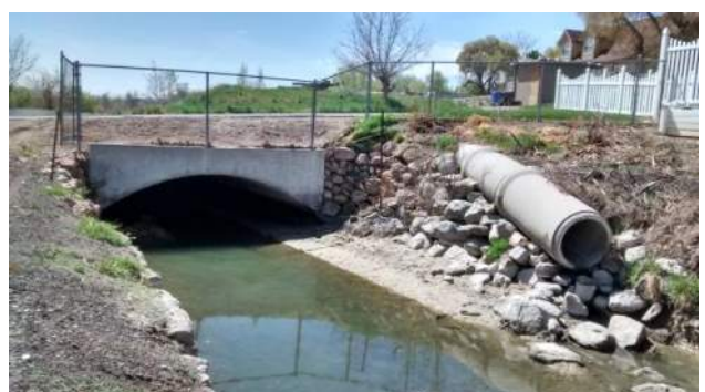
Culvert at Bennion Blvd. and 30 inch Outfall at Approximately 6235 South
