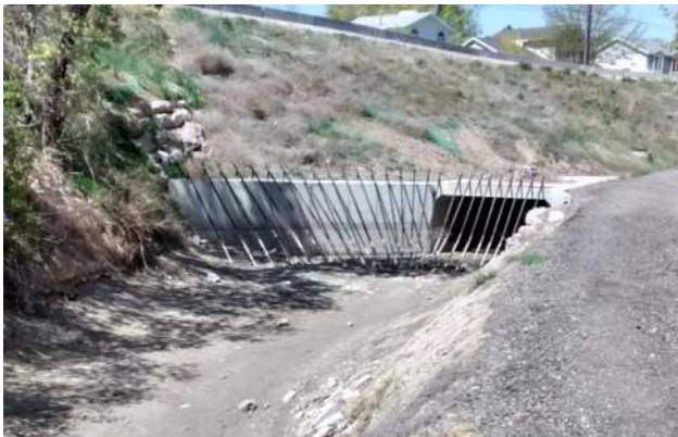
Trash Rack Upstream of Enclosed Canal at Approximately 5500 South
