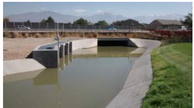
I-215 Overflow Structure
