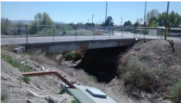
Bridge and Pump Station at Morning Sun Drive
