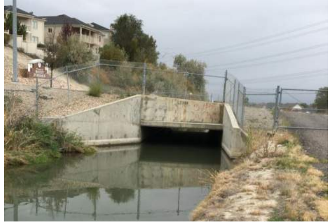
Culvert at 7200 South
