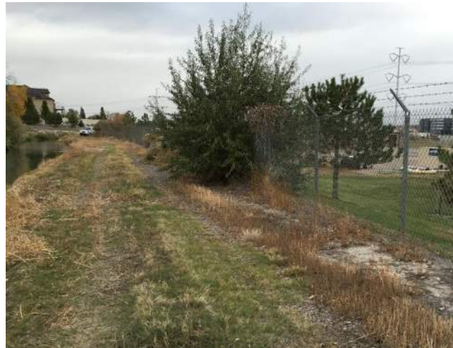
Tree in Embankment at Approximatley 7450 South
