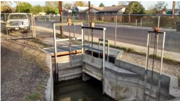
Outworks to the NJC pipe
