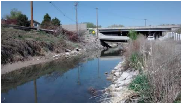
I-215 Overpass and Maintenance Access Bridge
