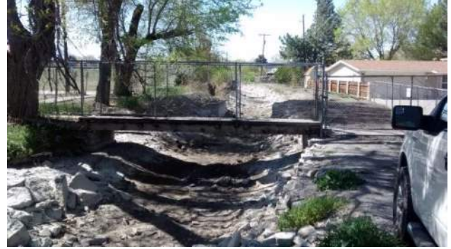
Footbridge at Approximately 2800 West
