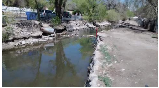
Outfall at Approximately 5850 South immediately upstream of I-215
