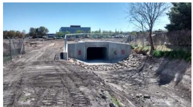
Culvert near American Express (Approximately 4240 South)
