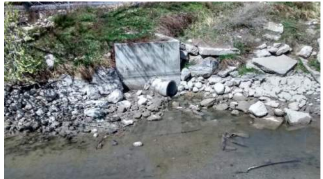
Outfall at Approximately 5770 South
