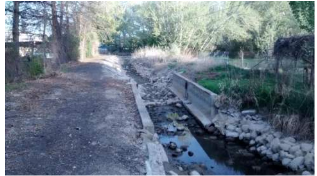
Concrete Flume Immediately West of 3200 West
