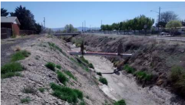
Pipe Crossing at Approximately 4950 South
