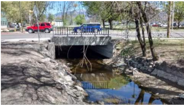
Bridge at 2200 West
