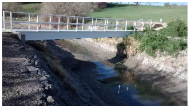
Pedestrian Bridge - Approximately 8250 South
