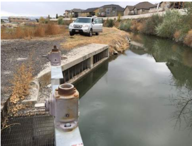
Storm Drain Overflow/Dump-out at Approximately 7200 South
