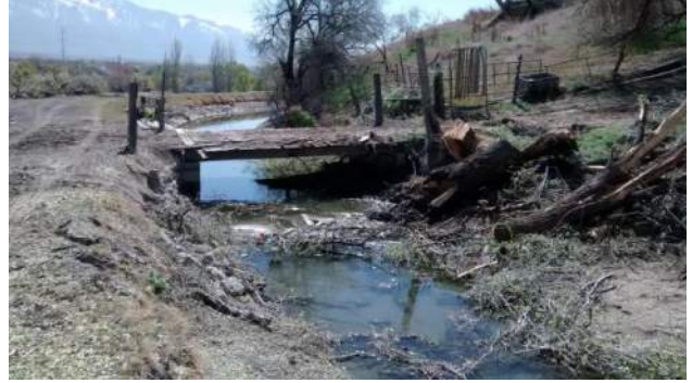
Wood Bridge at Approximately 6400 South
