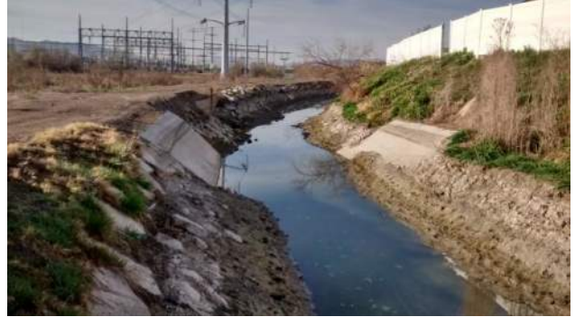
Utility Crossing – Approximately 8750 South
