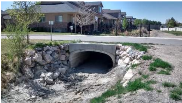
Bridge at 2290 West
