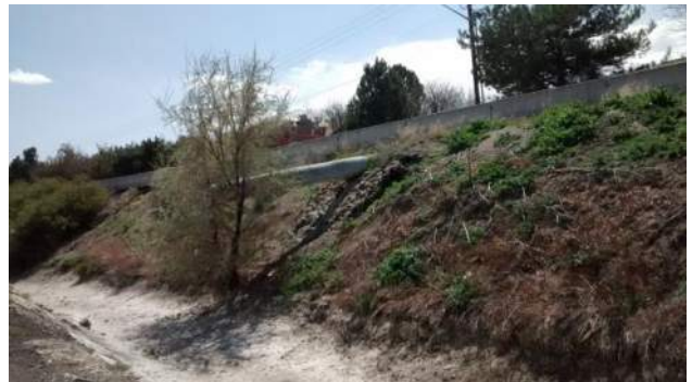
24 inch Outfall at Approximately 5350 South
