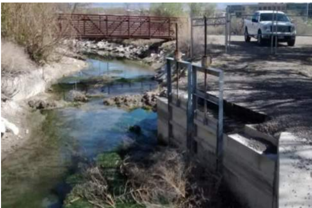
Storm Drain Overflow/Dump-out and Pedestrian Bridge at Approximately 7200 South
