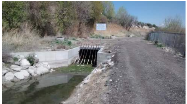
Trash Rack Upstream of Enclosed Canal at Approximately 6500 South
