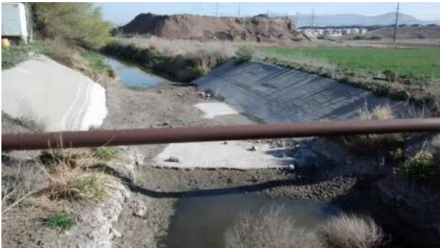
Bingham Creek Crossing – Approximately 8050 South
