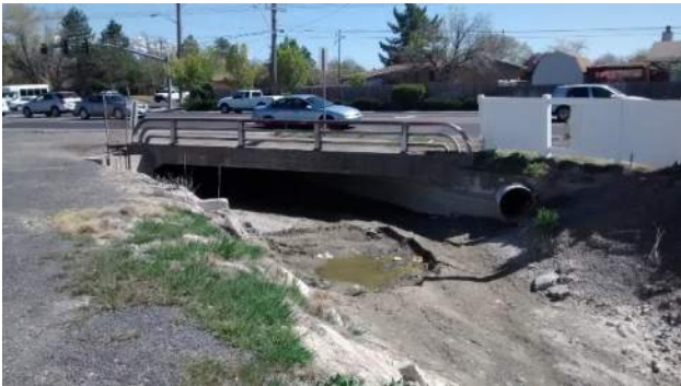
Redwood Road Bridge
