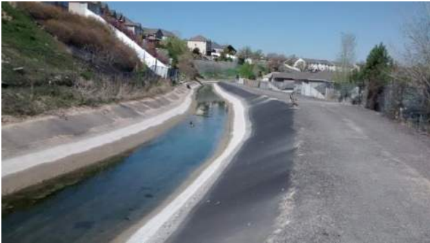
Canal Lining at Approximately 6700 South
