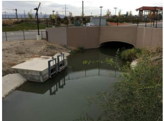
UTA Crossing and Storm Drain Overflow Structure Immediately South of 7800 South
