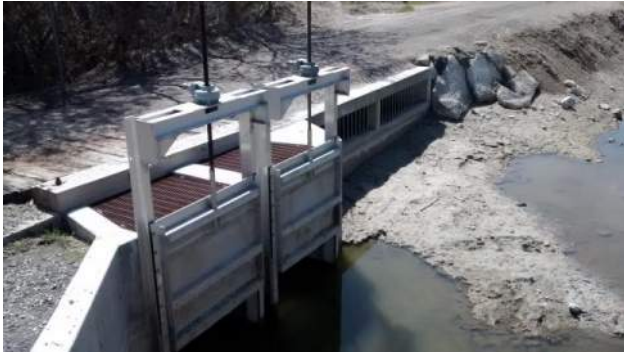
Storm Drain Overflow/Dump-out at Approximately 5600 South
