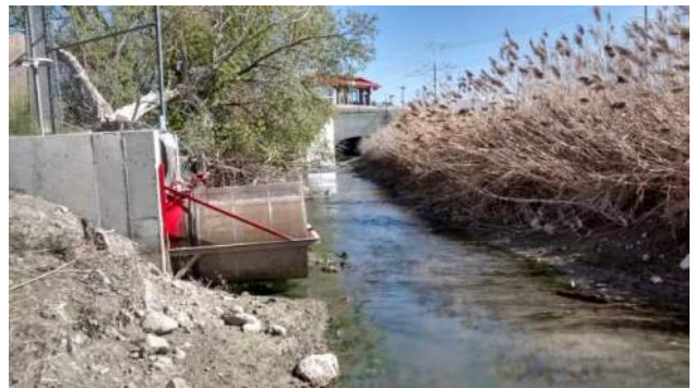
Pump Station Intake at Approximately 7600 South
