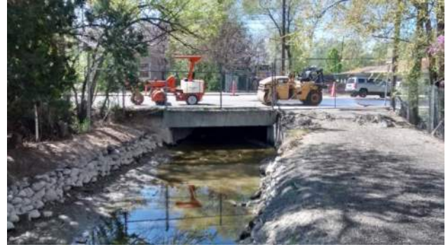
Bridge at 3200 West
